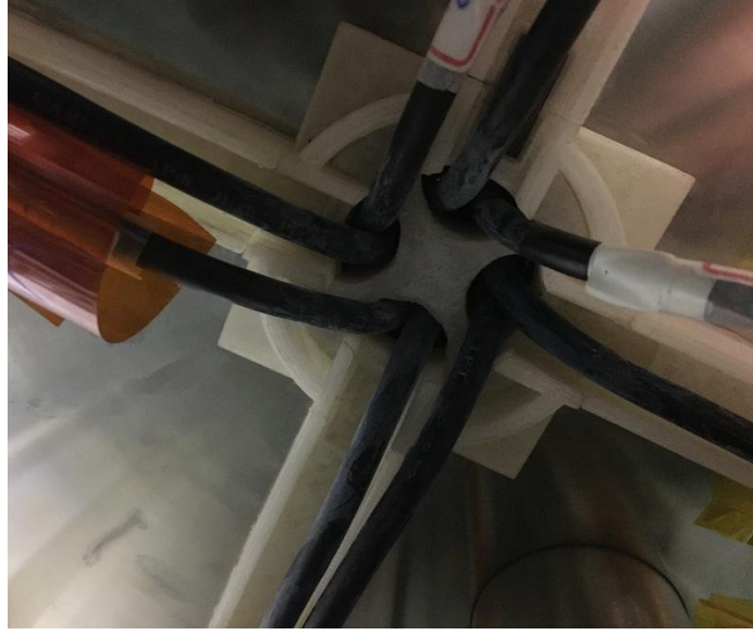
Figure 4.6: The eight turns toroidal magnetic field coils at tokamak bottom plate.
